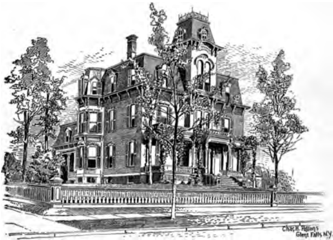
Residence of Gen. William Wells, South Willard Street.
